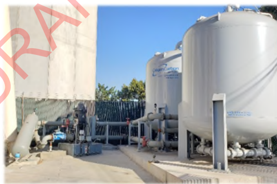
Figure 2.4: TCE and GAC Treatment at Well 15
