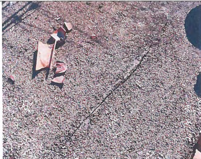
Photo 7: Split at Section B
